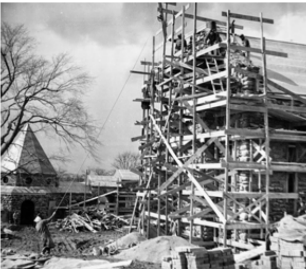
Construction of the new monastery.
